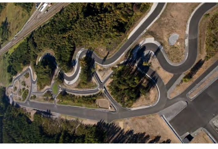
Arlanda test track
